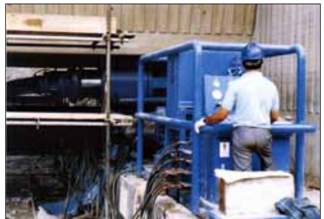
Above: L600 jacks and L4/15D powerpack performing a launch.
