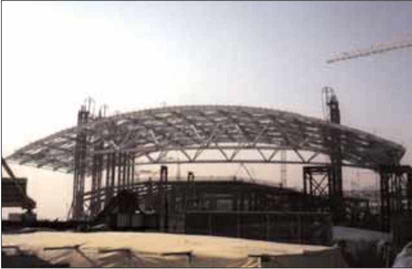
Above: The largest truss, weighing 1250 tonnes, in it's final lift position.
