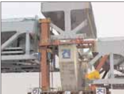
Left: Jacks can be seen climbing up the cables.
