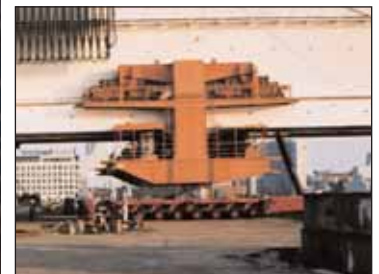
Below: The main girder lower crane trolley (160 tonnes) being lowered onto an 8 axle Fagioli SPMT
