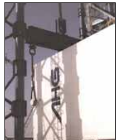
Above: Fixed anchor housing with swivel and spreader beam arrangement.
