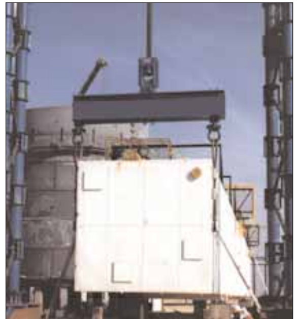
Above: Fixed anchor housing with swivel and spreader beam arrangement.
