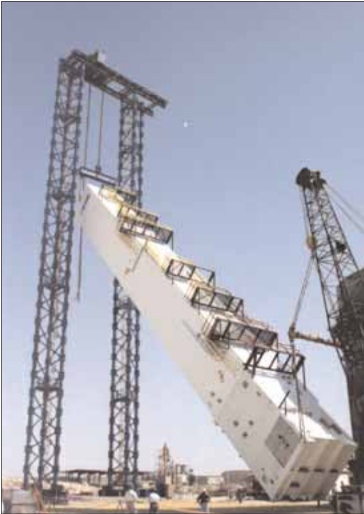
Above: Fixed anchor housing with swivel and spreader beam arrangement.
