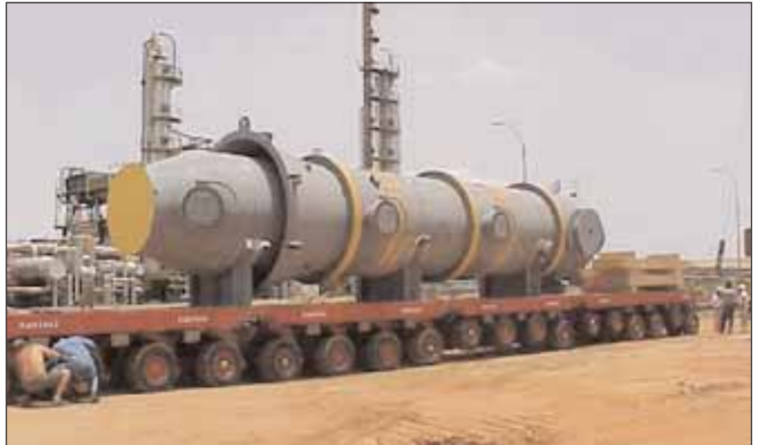
Above: One of the components arriving at Tema Refinery
