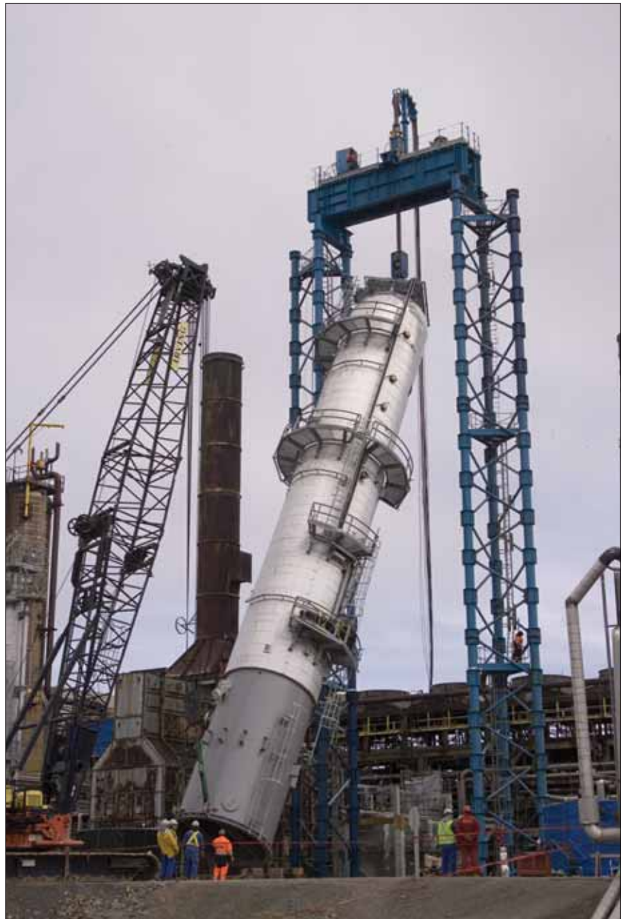
Above: Reactor being lifted by Fagioli PSC Tower system
