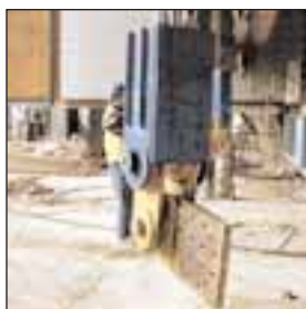
Above: An adaptor plate with a pin connection to the blue L100 fixed anchor housing.
