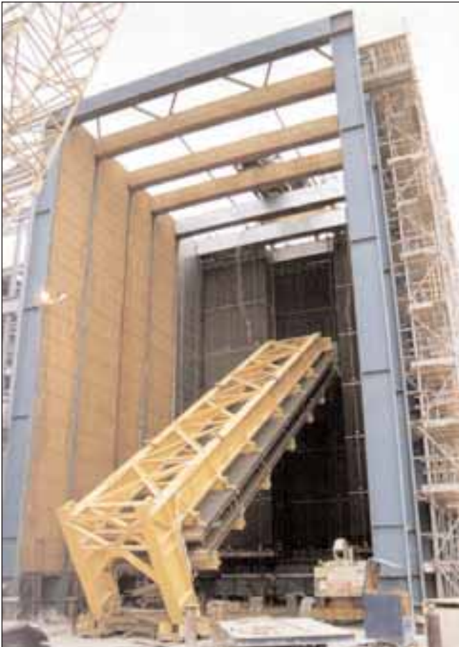
Above: a module in its 'strongback', half way through a lift.
