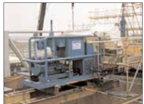
Below: L4/15D power pack and two L100 jacks on their mounting beams.
