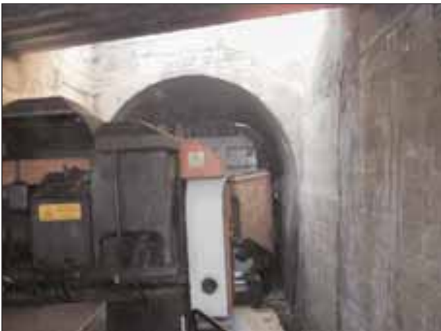
Below: The extremely tight Buschdorfer Tunnel
