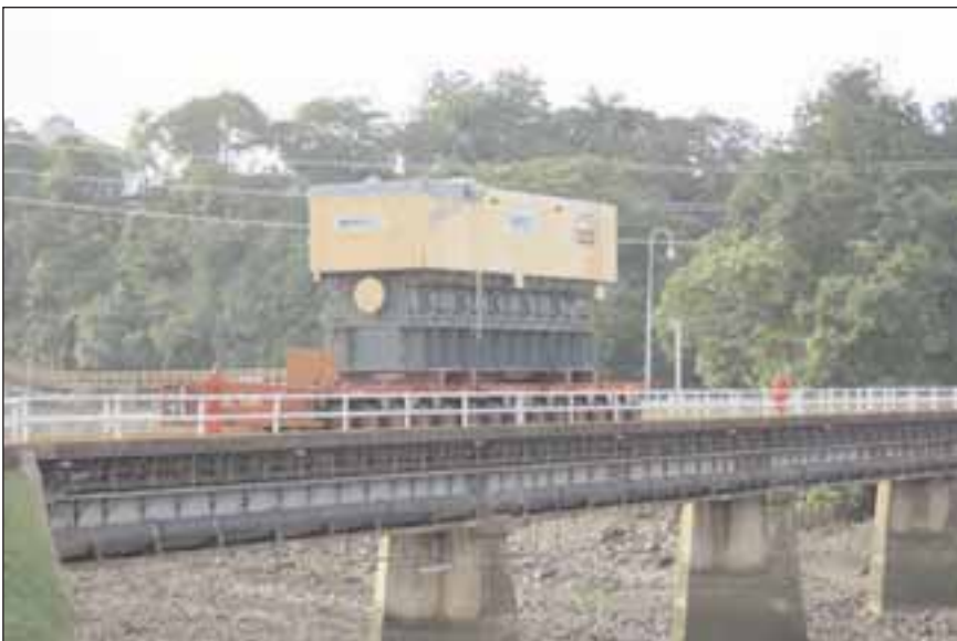
Above: Crossing over the Bridge built in 1901
