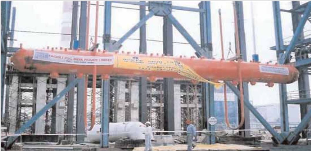
Left: Initial view of boiler drum
